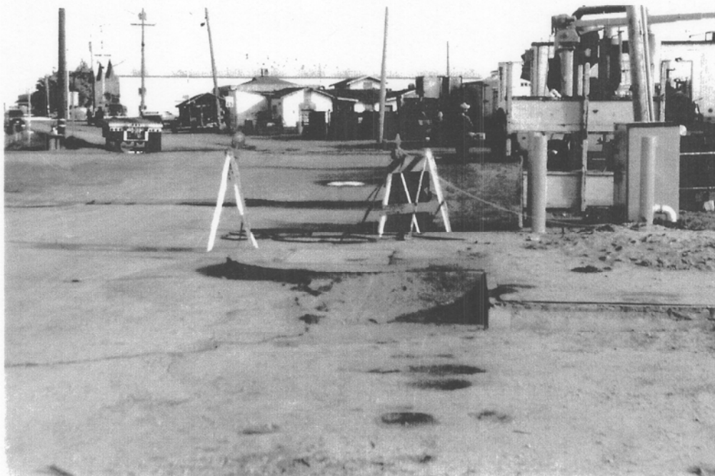
FIG. 8-2(a). Differential Settlement at a Sewer Well on Sandholdt Road, Just to the North of the MBARI Pier (looking north).
