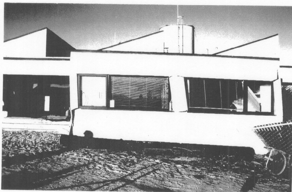
FIG. 9-2(b). Racking of Southern Building at Southeast Corner of MLML.
