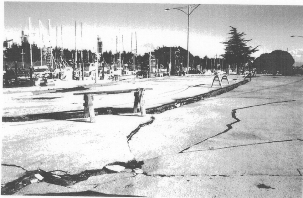
FIG. 6-3. Cracking at North End of Parking Lot Near Dock "C."
